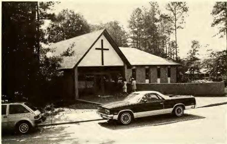
First building which was completed in November, 1975.
